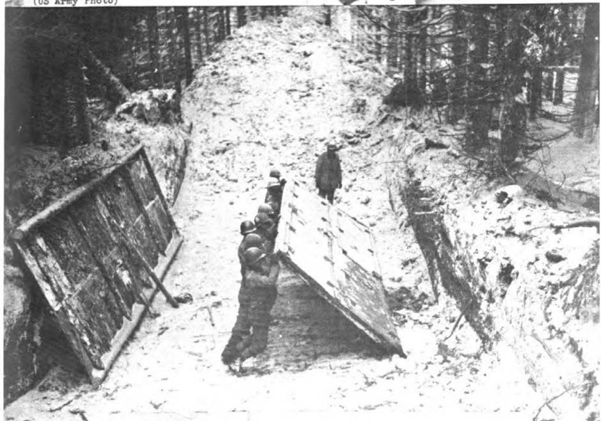
Men of the 324th Engineers put up the side wall of a dugout in the Rehabilitation area. (Co 'B' 324 Engrs)
